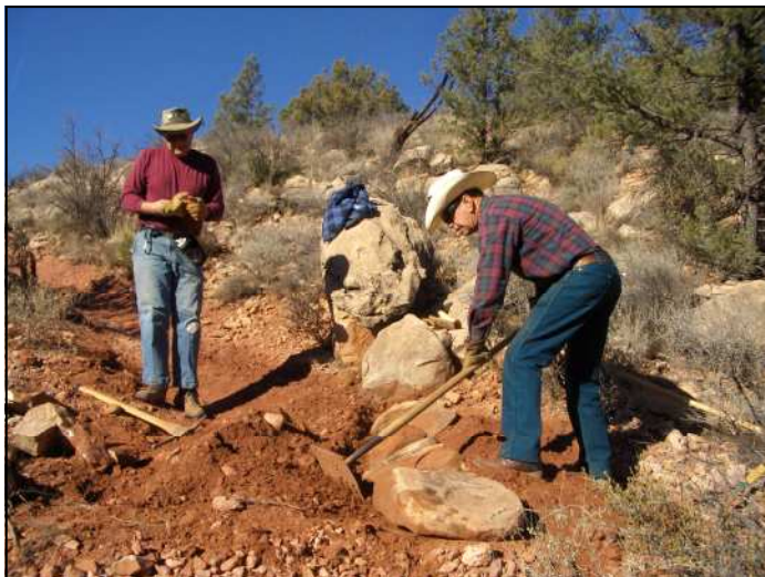
Kevin Harding and Gene Rector constructing a rolling dip on Carroll Canyon Trail.
