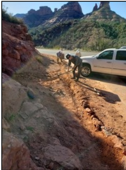
Midgley Bridge Drain
