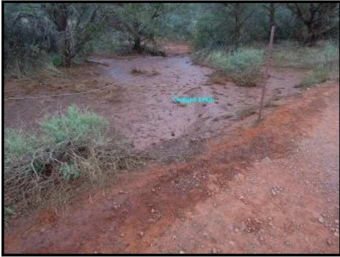
Culvert drains clogged with mud and debris on Bell Rock Pathway
