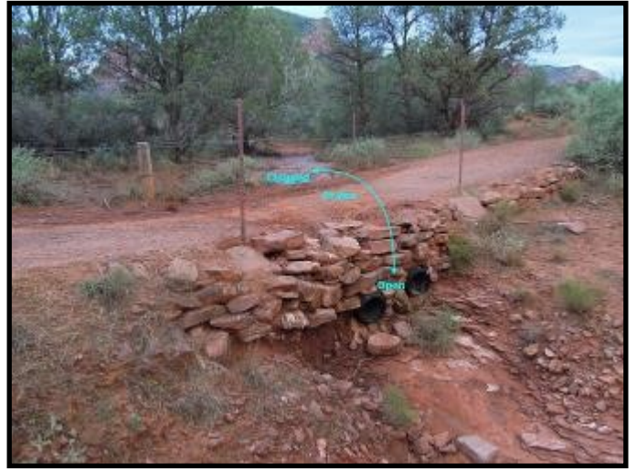
Culvert drains clogged with mud and debris on Bell Rock Pathway
