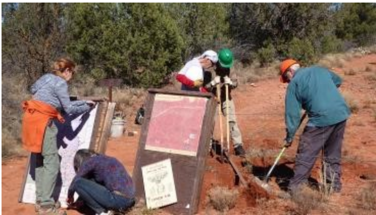
Post holes being dug and aligned before placing new Kiosk. Pictures by Jean Ober
