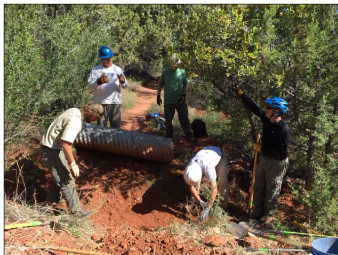
Culvert installation on Allen's Bend trail!
