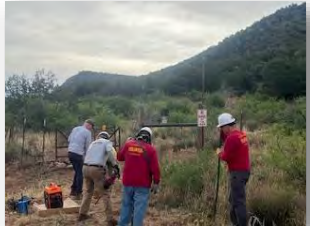
Preparing the Ground at (the other) Long Canyon
