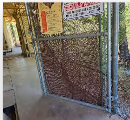
Repaired access gate
