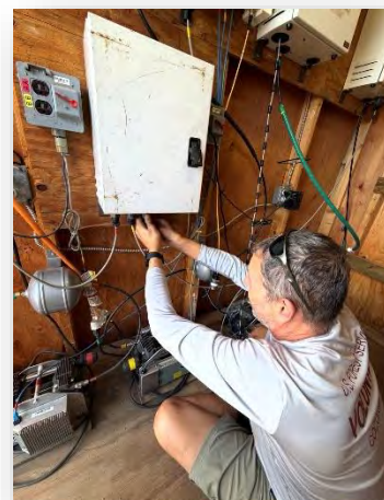
Jerry Checchia repairing equipment
