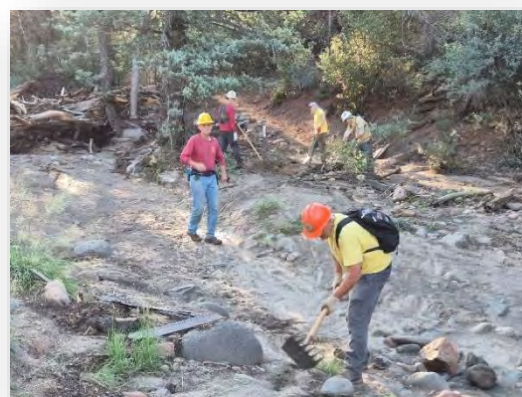
The FOF crew repairing the AZ Cypress Trail
